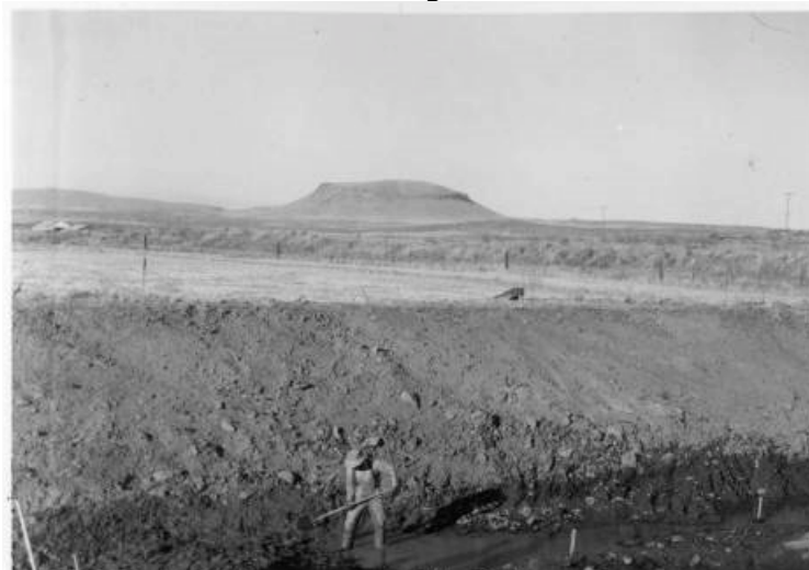
View looking north showing excavation for pumping plant. Rock in drain has not been removed to grade; October 21, 1958; Photo by K. J. Greene
